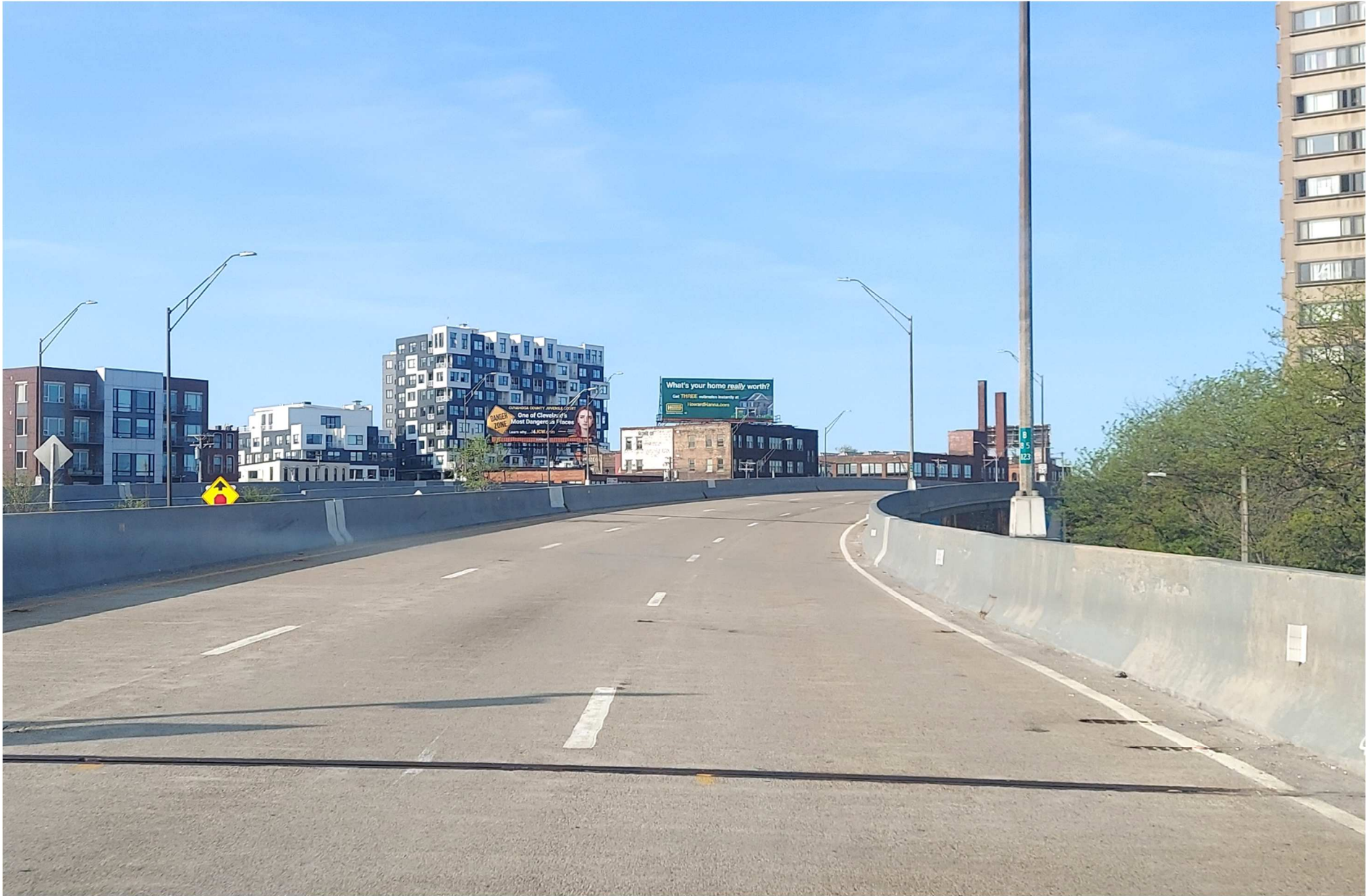
Figure 34: Photo of existing Shoreway in Ohio City looking west
